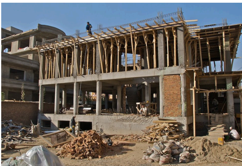
A previously destroyed building undergoing reconstruction with concrete reinforcement. 104
