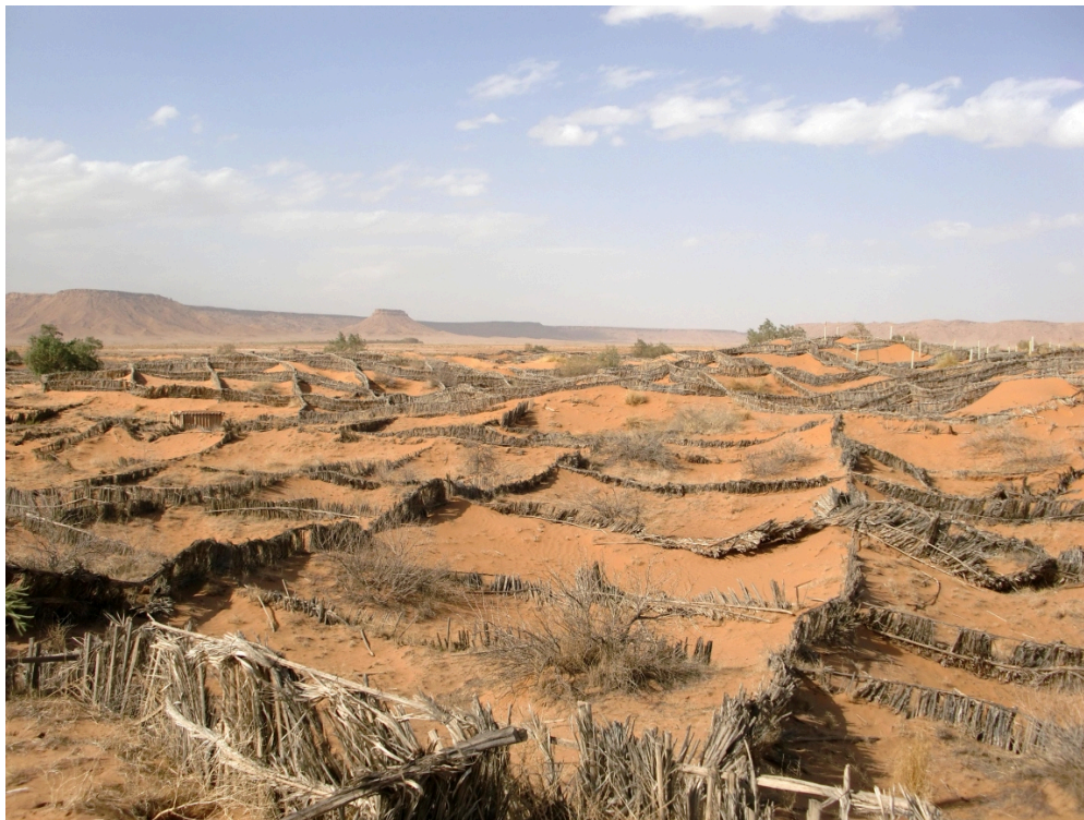
Sand fences to combat desertification in Morocco. 95
