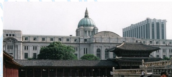
Figure 7. Japanese General Government Building in Seoul, South Korea 83
