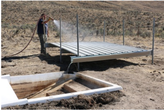
Volunteers help build wildlife water tank (Bureau of Land Management, 2015)
